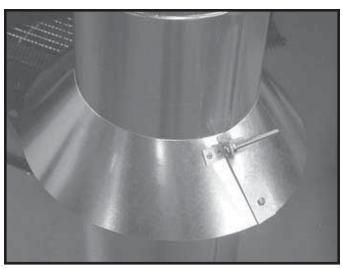
Figure 8.20 Assembling the Storm Collar Around the Pipe
